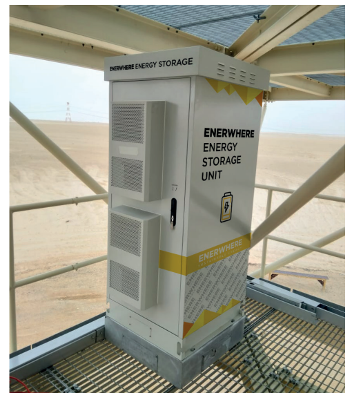
Energy storage unit in the tower.
